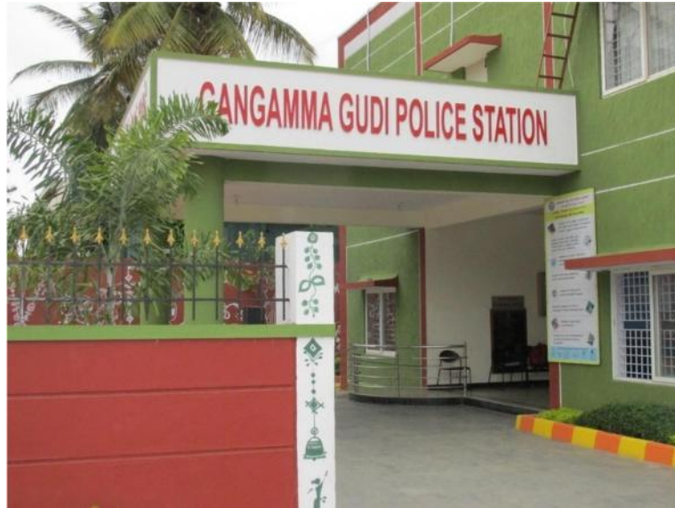
Figure 101: Gangamma Gudi Police Station Building
