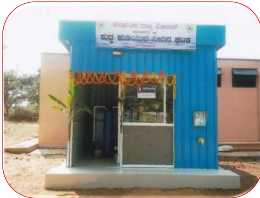
Figure 40: RO Water Purification Plant at Chikkaballapura
