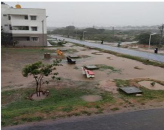
New Police Quarters, Basapura Village
